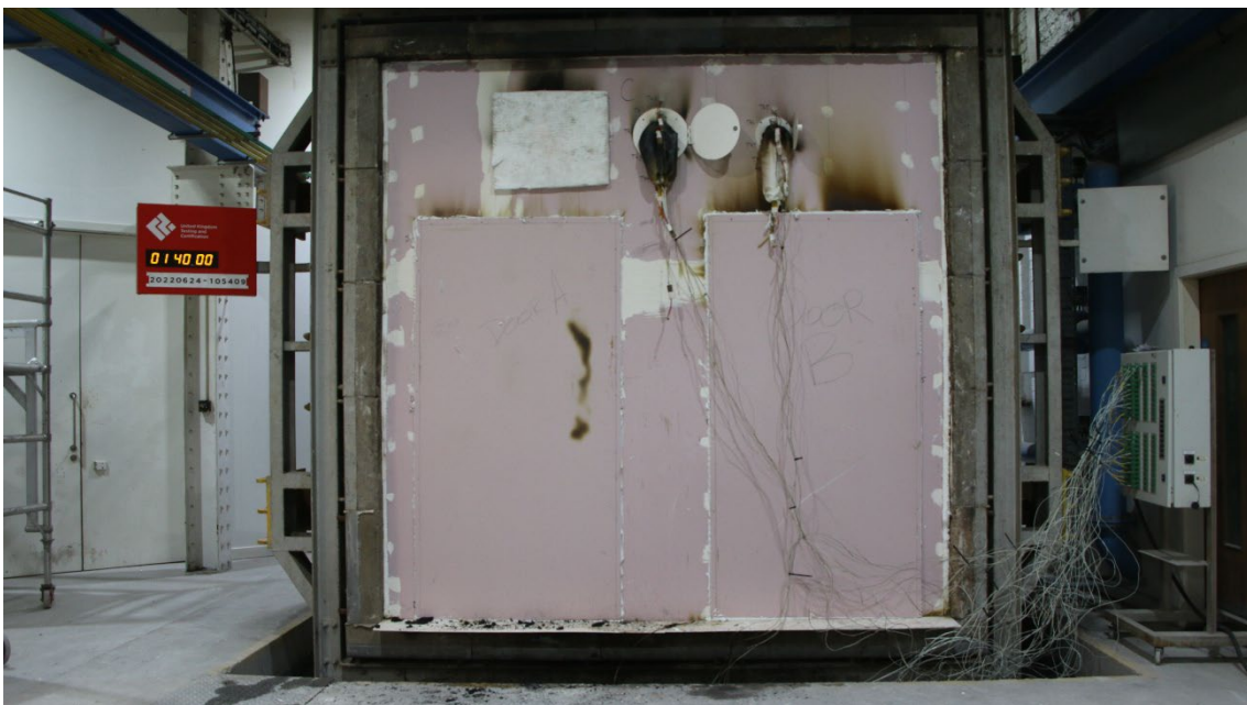
Figure 28 - The unexposed surface of the test construction after a test duration of 100 minutes
