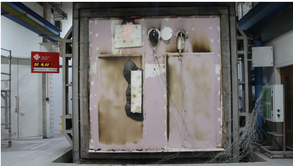
Figure 32 - The unexposed surface of the test construction after a test duration of 136 minutes
